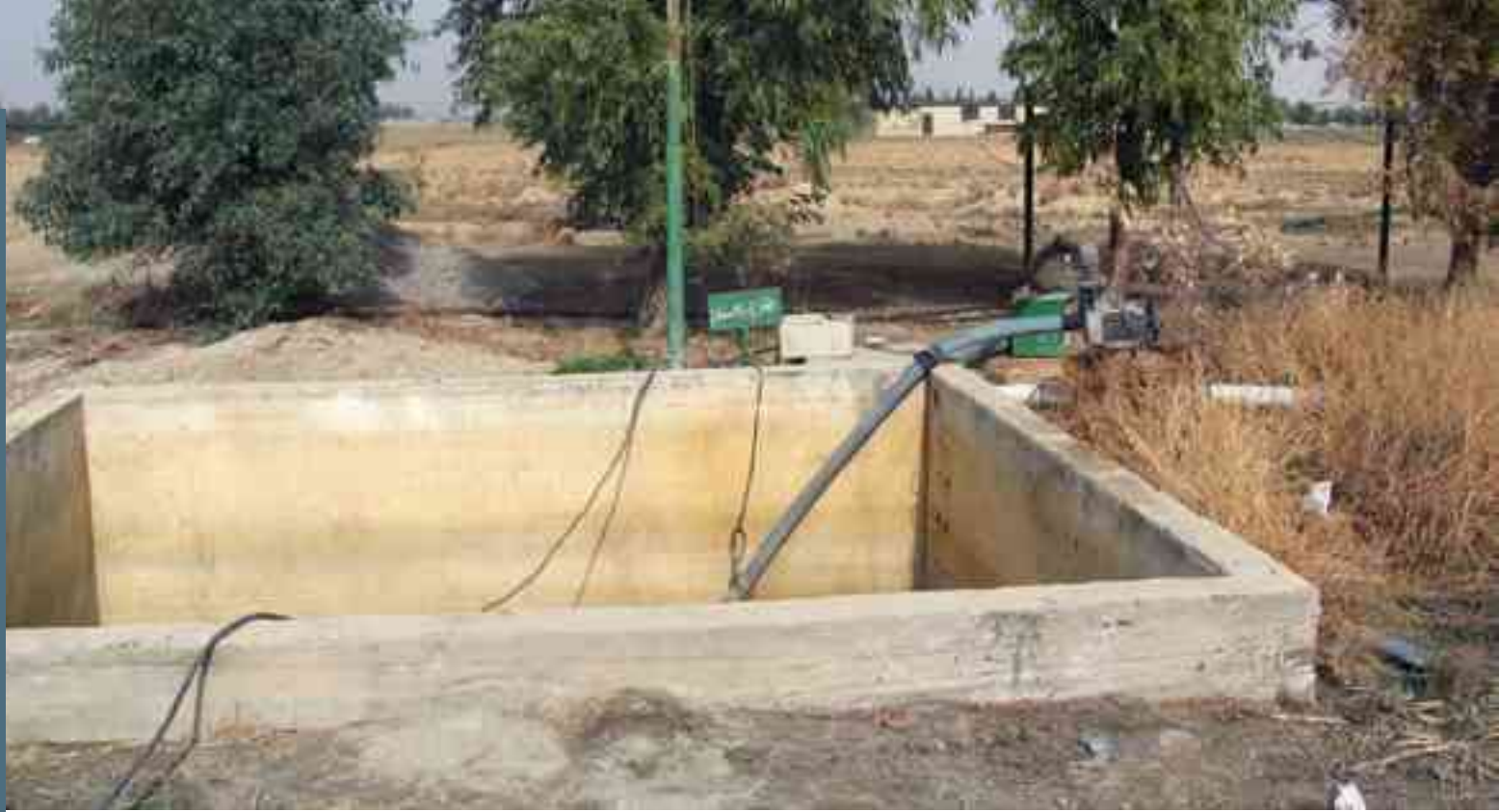
Storage tank from which treated effluent is pumped for irrigation at Haran Al-Awamied, Syria. Source: SuSanA Secretariat
