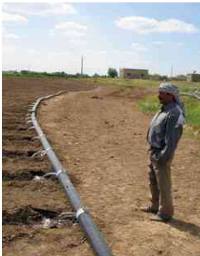
Modernized on-farm irrigation system in Syria: an example of a gated-pipe.
